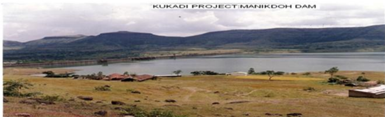
Photo No.02 – Kukadi Project On Manikdoh Dam
